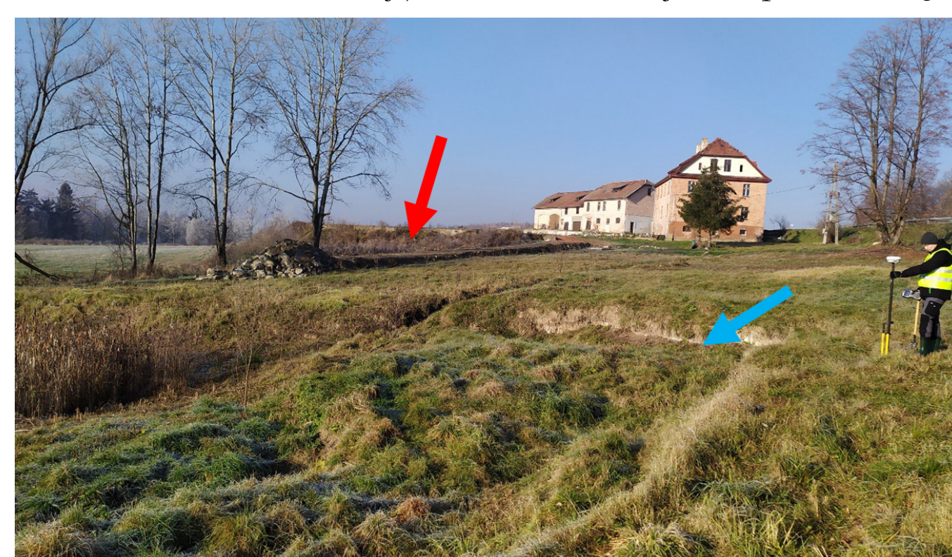
Fig. 3. Photographic documentation of the displacement line directly in the culvert zone under the district road No. 2491D, km 18 + 739.85 - 18 + 836.17 (on the left) and the sub-areas of the asphalt roadway deformation (subsidence troughs visible as light yellow areas).
