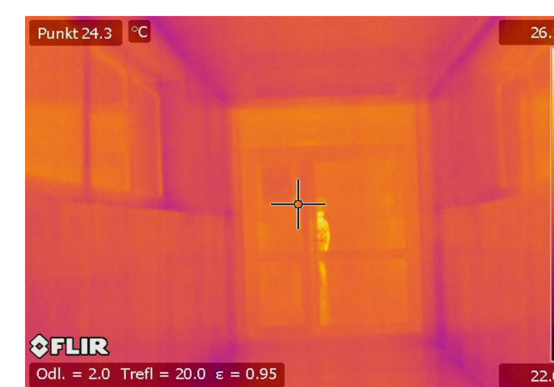
Fig. 8. Temperature distribution inside connector No. 1
